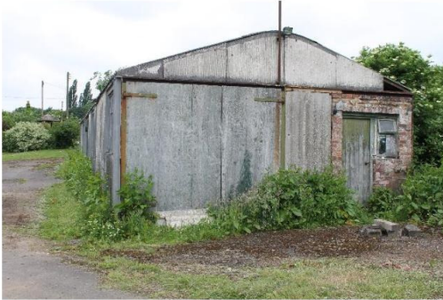
Existing building east facing.
