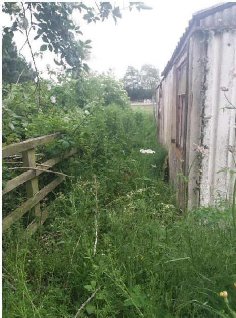
Existing building and boundary north side
